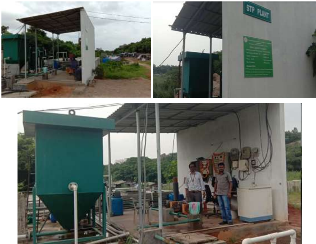
Sewage Treatment Plant (STP) setup within the Campus
