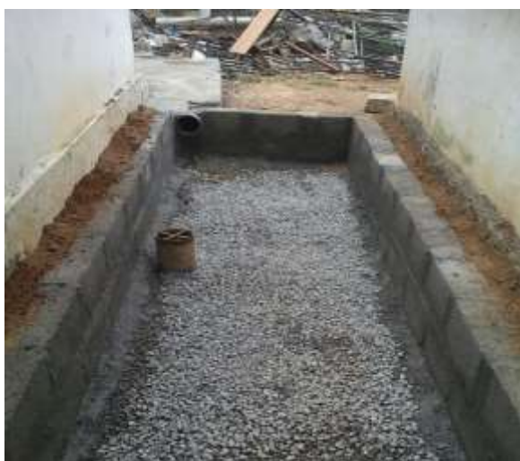
Borewell Recharge Pit and recharge pit through Soil Bund
