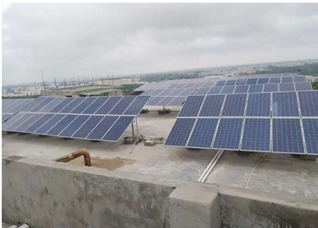
Solar Plant and Solar Streetlighting availability in the Campus
