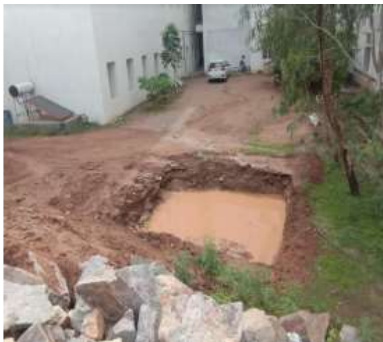
Rainwater Harvesting Percolation Pits
